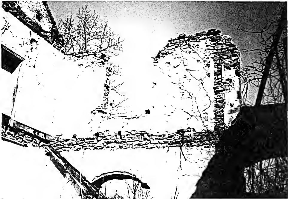
Figure 32: Interior view of window along east elevation
